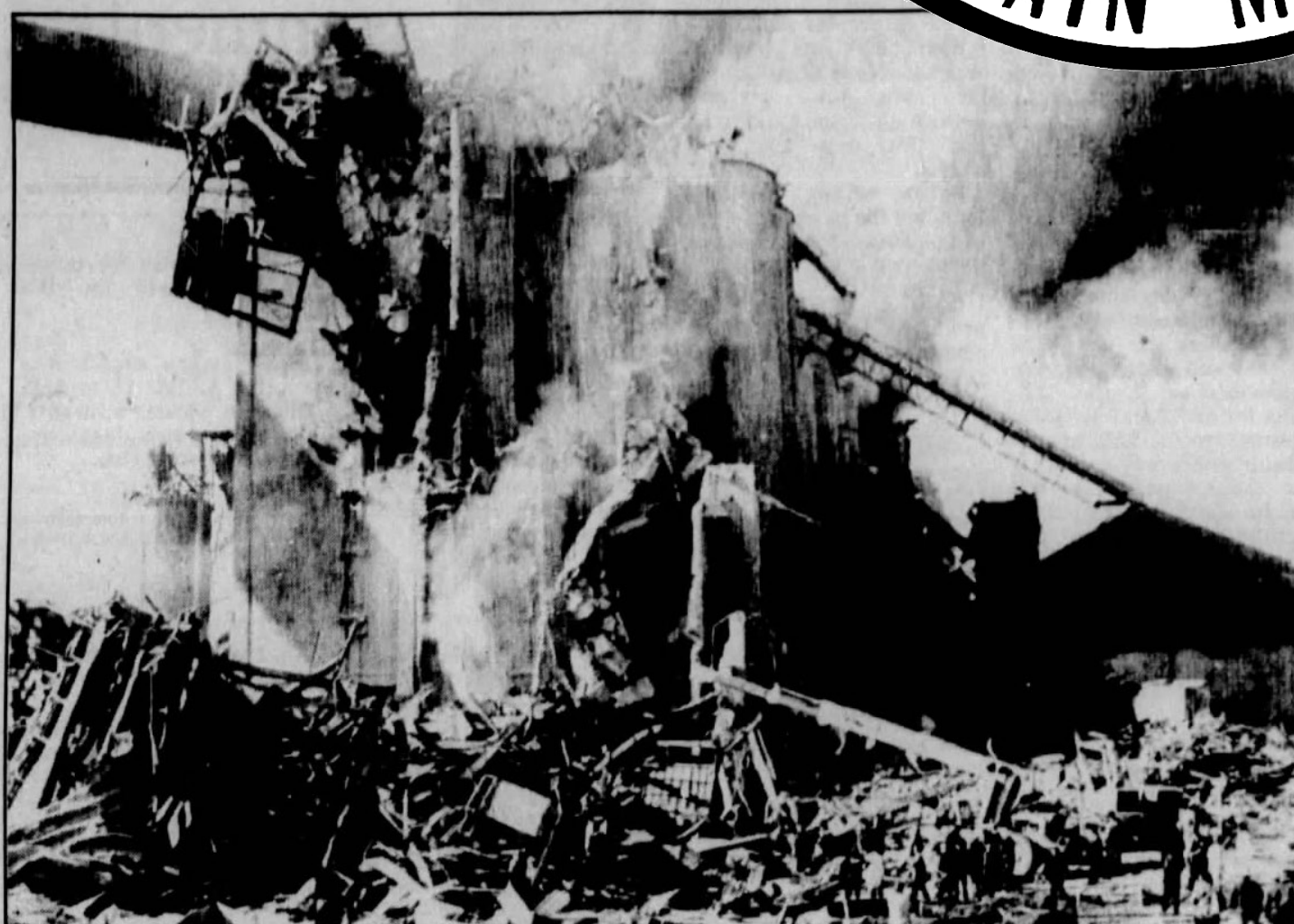
This is the scene of a Continental Grain elevator explosion Dec. 22, 1977, in Westego, La.
