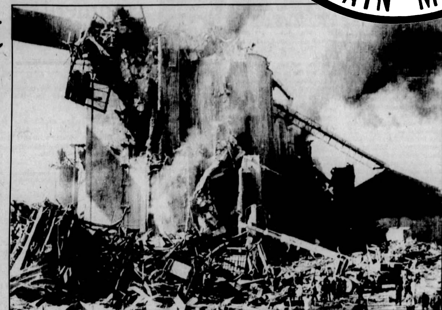
This is the scene of a Continental Grain elevator explosion Dec. 22, 1977, in Westgo, La.
